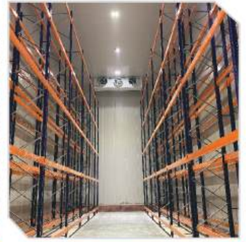
Double deep Pallet Racking
