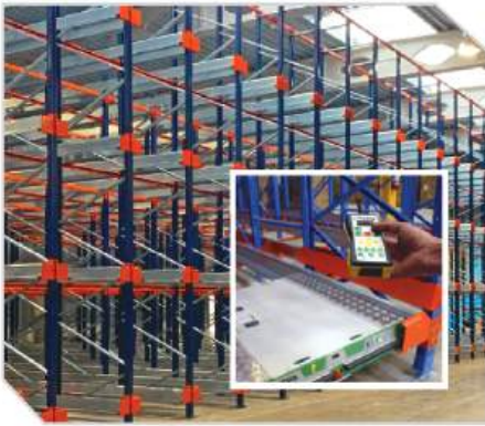
Shuttle Pallet Racking
