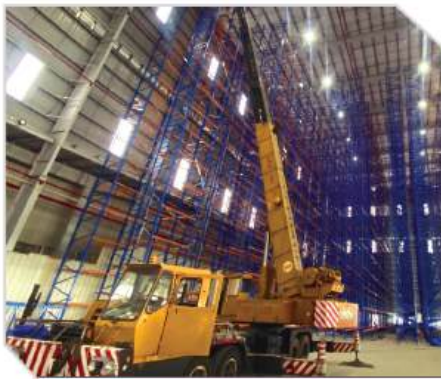
Dismantling and Reinstallation
